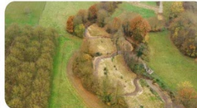
Remanufacturing of the Herbasse river in 2018 (Photo credit: SIABH)
